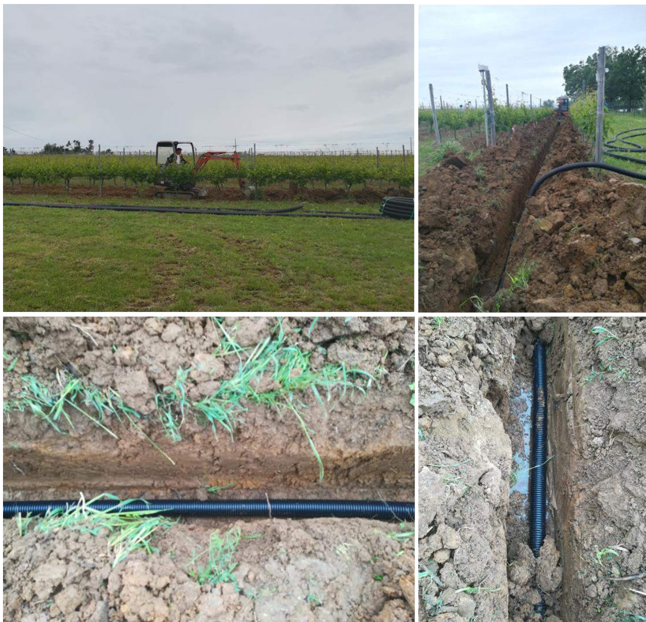
Figure 38: Drainage installation in RES1 demonstrative vineyard
