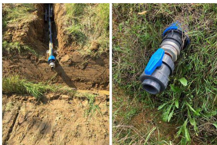
Figure 39: Particular of the final tap of the drainage RES1 demonstrative vineyard
